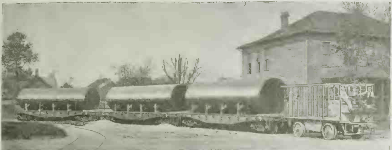
An Electric Truck "Doing Its Bit" Somewhere in New Jersey. This Truck, Equip with Edison Storage Batteries, Is Hauling Three Tank Cars Without a Whimper.
